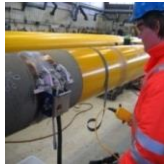
Inspection (NDT) and Quality Control
